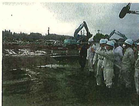
(益城町既存仮置場)
